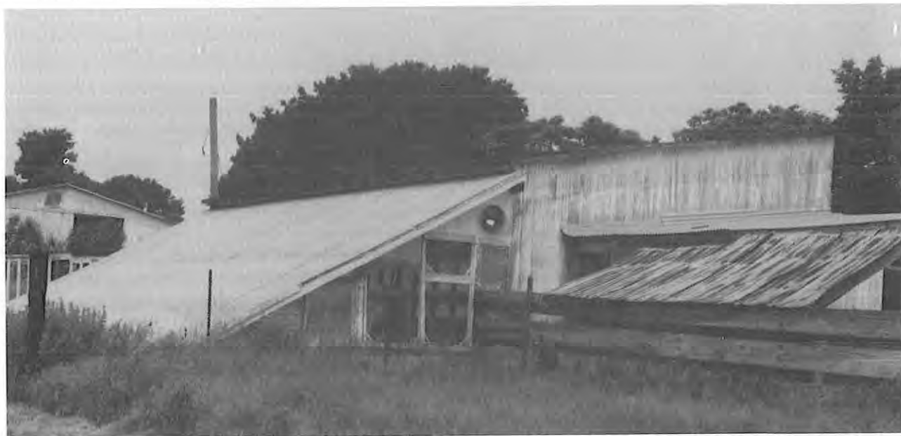
Wayne built a lean-to greenhouse on the south side of a large barn to use in early spring for propagating the various crops produced on his farm. He uses a wood frame and chicken wire shelter for starting crops and bedding plants. This structure helps to protect the tender young crops from bird and animal damage.
