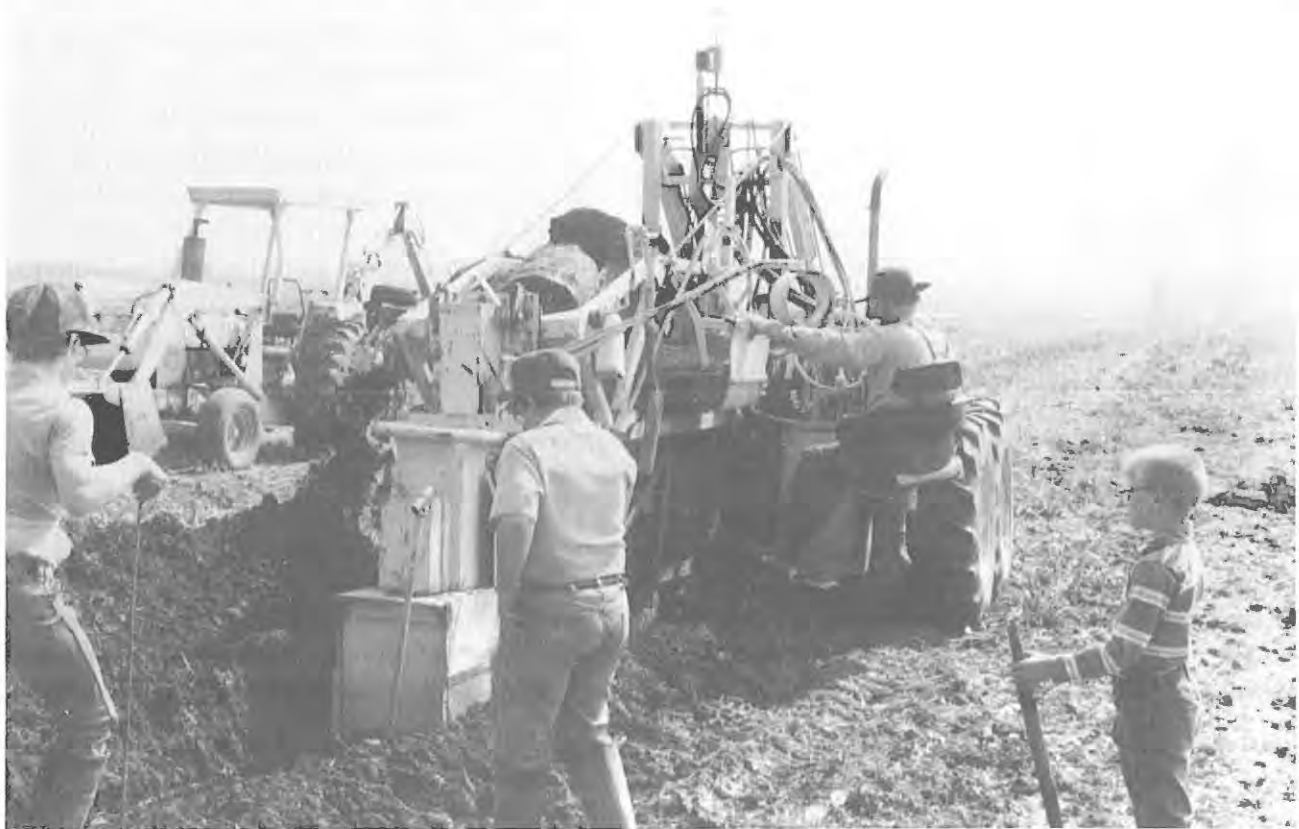
Carl's ditching and tiling services are in constant demand because much of the relatively flat farm land in his area would be impossible to till without proper drainage. Carl repairs existing drainage systems in addition to installing new drain tile. His children often assist with the repair and maintenance of equipment, and under Carl's close supervision, sometimes help at job sites, as well.
