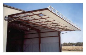
allow the operator to pull on a vertical rope rather than push or pull on a sliding door. Using wireless or remote controls to activate power door openers can reduce the need to mount/dismount equipment when accessing storage areas. A wide range of automatic door openers for farm applications are commercially available.
