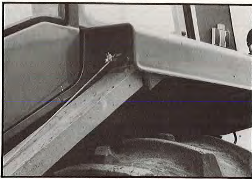
Figure 9. Cable attached to Steel Channel
