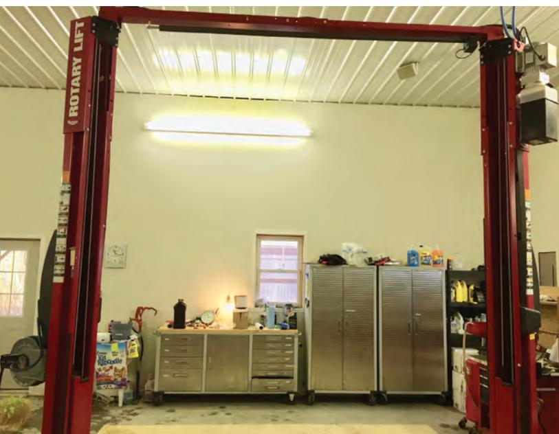
*Figure 4. Wall-mounted lighting provides both top-down reflected light and side-angled light, resulting in less perceived shadows on work areas.*
