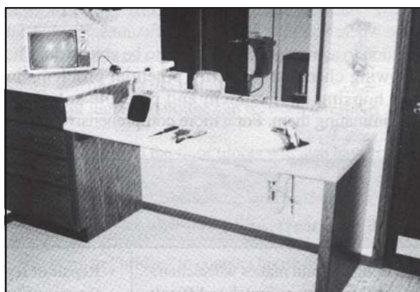
Figure 3. A lowered roll-under countertop in the bathroom provides easy access to sink and mirror. Note faucet placement on side of sink. A roll-away cart could also be used under the counter for additional accessible storage for toiletries, make-up, towels, etc.
